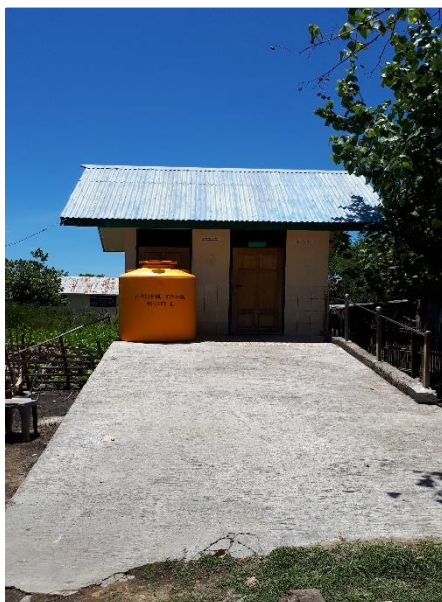
Figure 10. MHM Toilet at the Intervention Primary School in NTT
