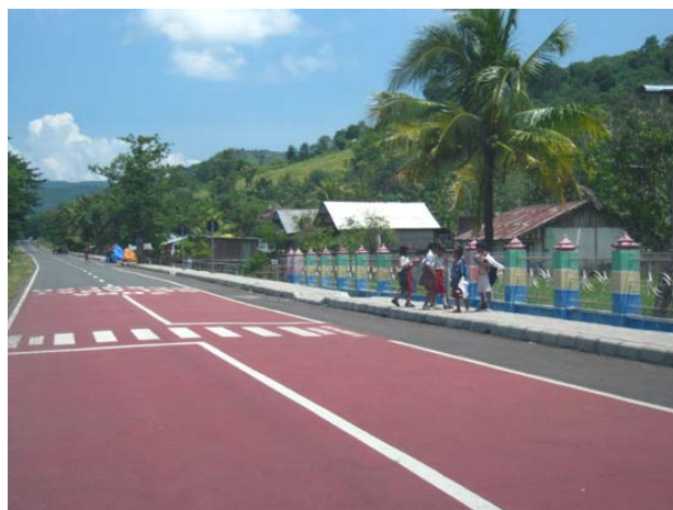
Figure 5. A photograph of a road in front of a school with a zebra crossing, sidewalk, and school safety zone (in red) following road improvement work by EINRIP.
